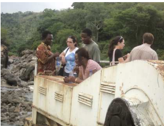
The MCC and MCA-M team at Tedzani Hydro-power station
